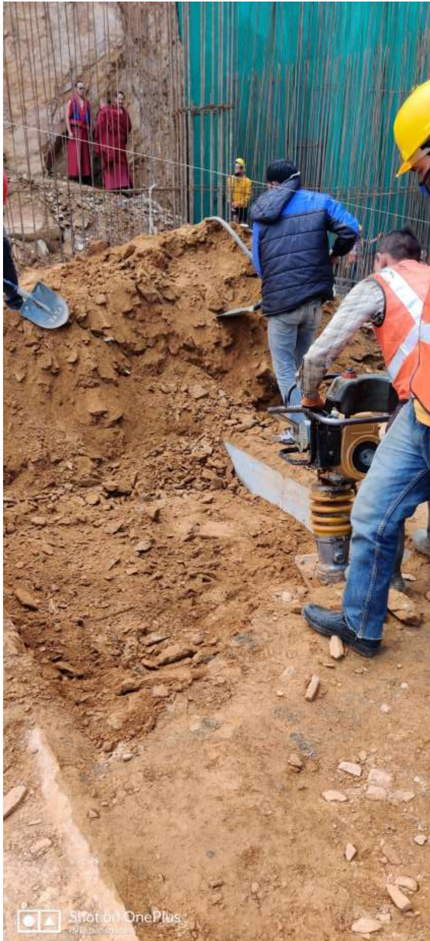
Picture 4: Back Bill and Earth compaction upto plinth level
