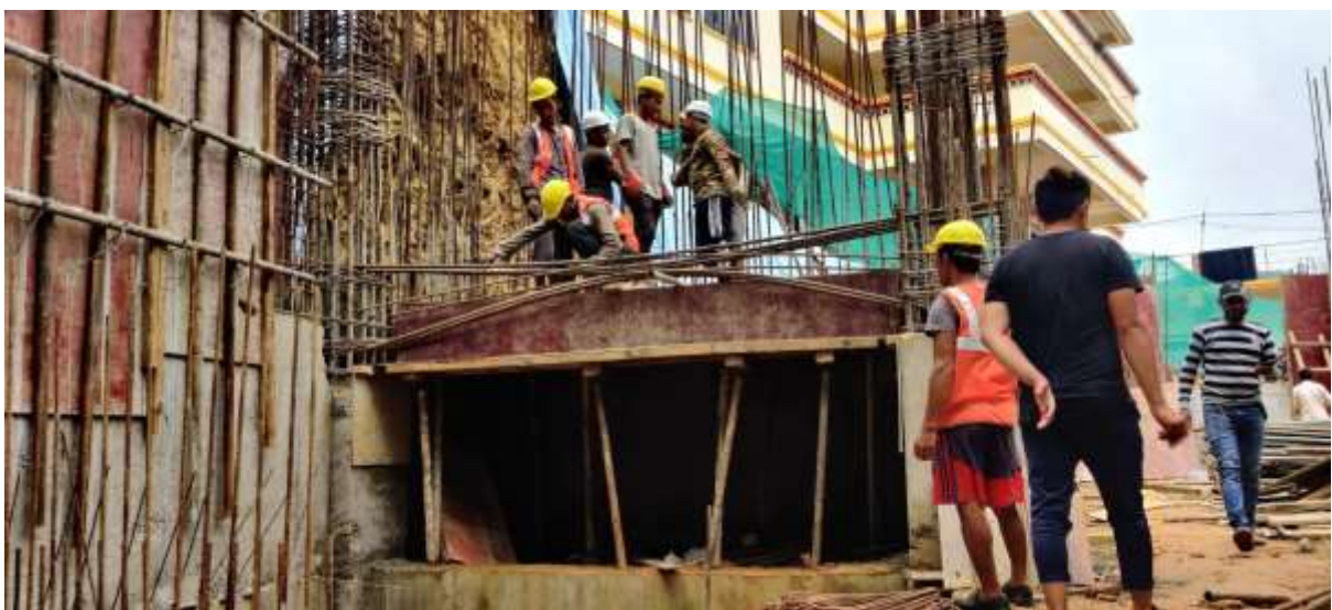
Picture 14: Rebar work at staircase landing
