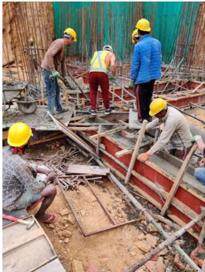
Picture 8: Concreting of Lower level Plinth Beam from Grid 1 to Grid 5
