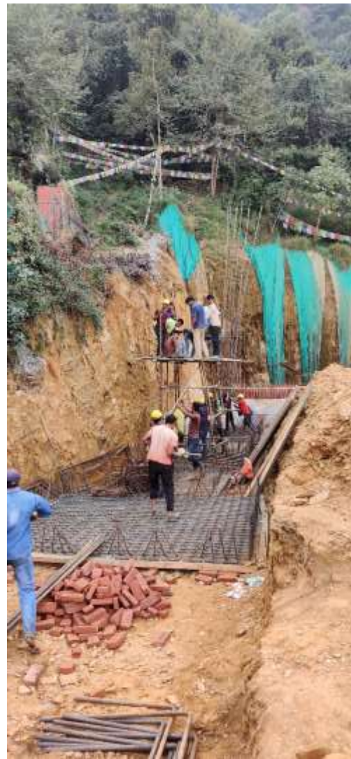
Picture 29: Rebar work for Upper Ground level foundation
