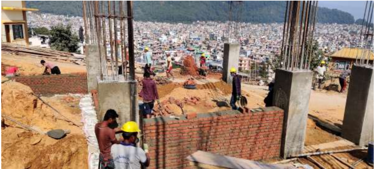
Picture 34: Brick Masonry work at lower ground level upto plinth level
