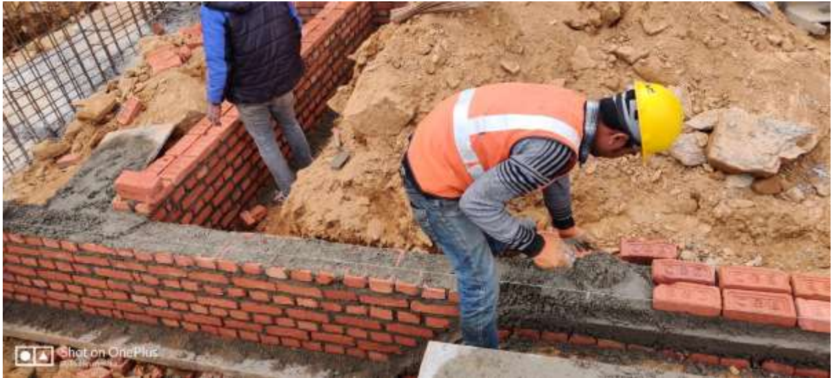
Picture 1: Brick Masonry work at Sub-structure
