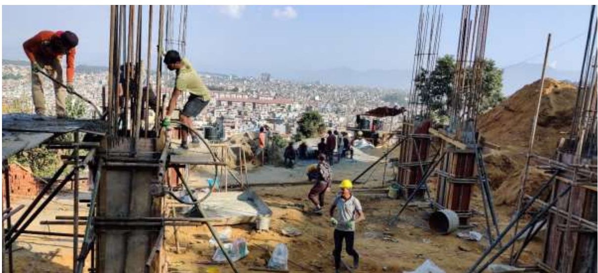
Picture 33: Concreting of lower level column upto Plinth level
