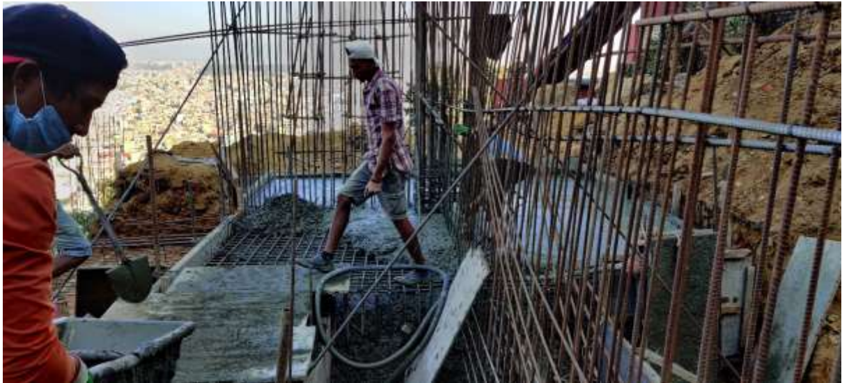
Picture 31: Concreting of Upper Ground level foundation
