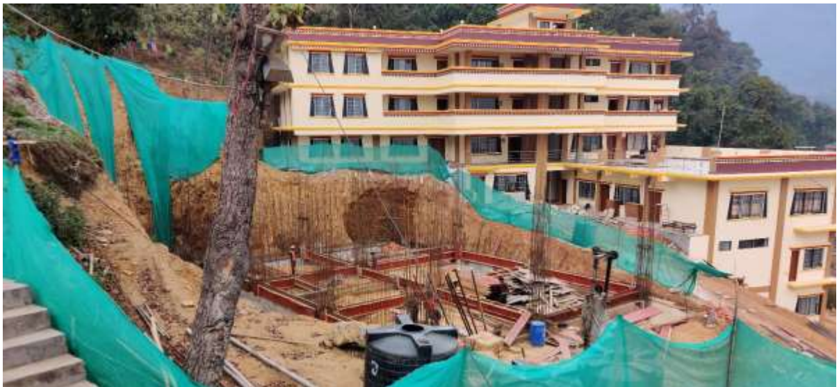
Picture 6: Formwork for Lower level Plinth Beam from Grid 1 to Grid 5
