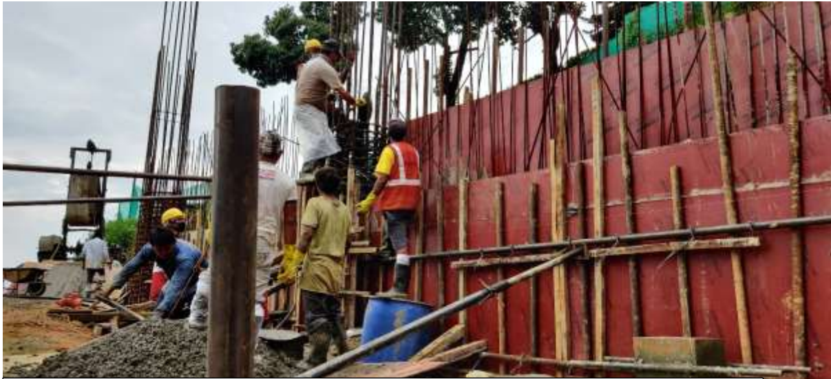
Picture 9: Concreting of Lower Ground Floor shear wall upto half Floor
