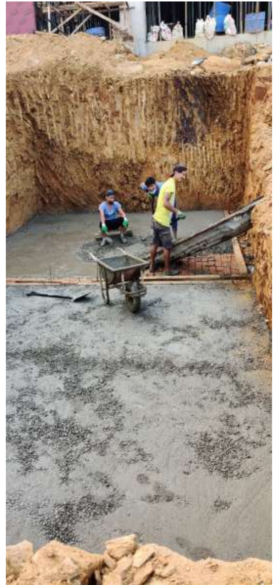
Picture 25: PCC for Foundation CF3
