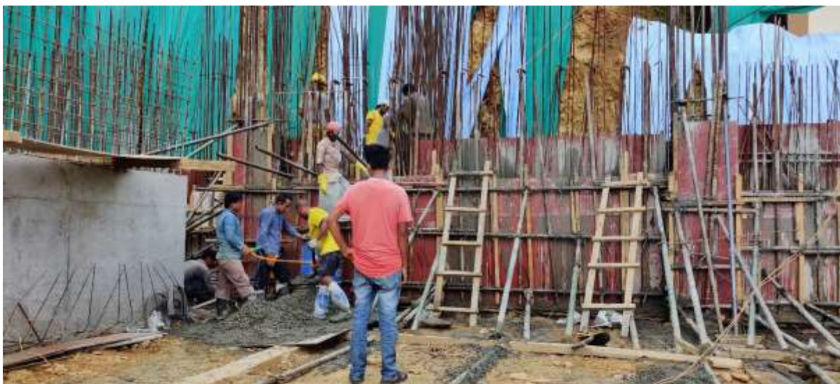
Picture 11: Concreting of Lower Ground Floor shear wall upto half Floor
