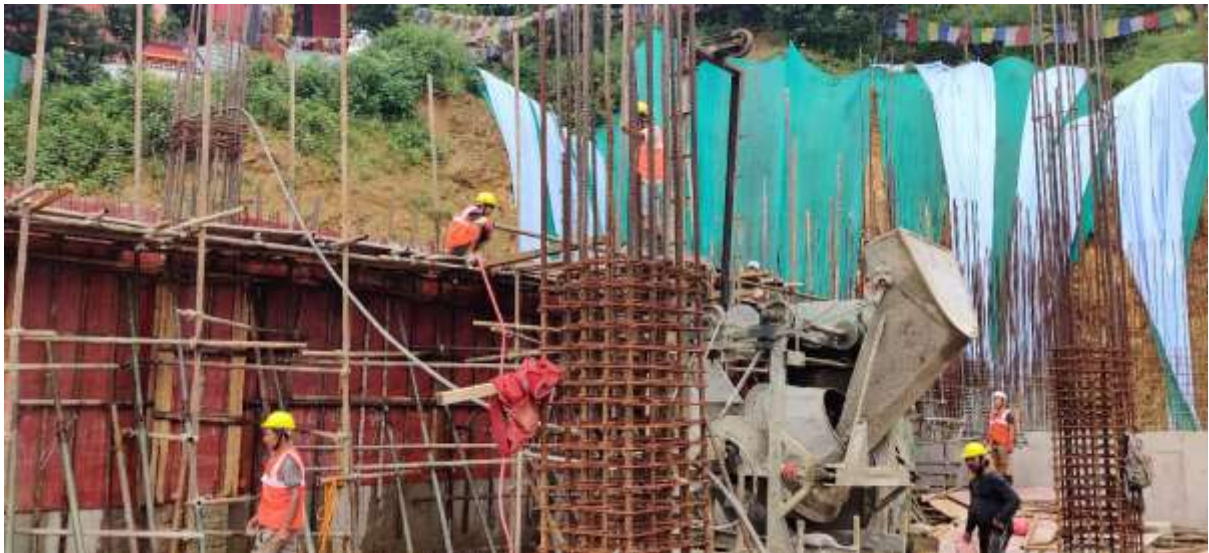
Picture 13: Concreting of Lower ground floor Shear wall upper half part
