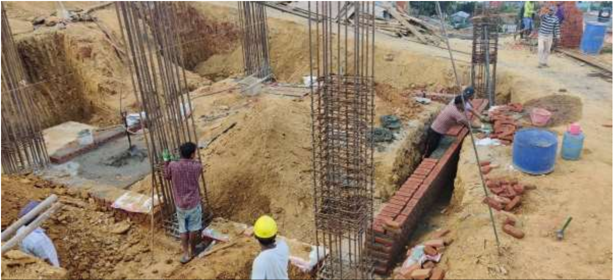
Picture 27: Brick Masonry work at lower ground foundation beam level
