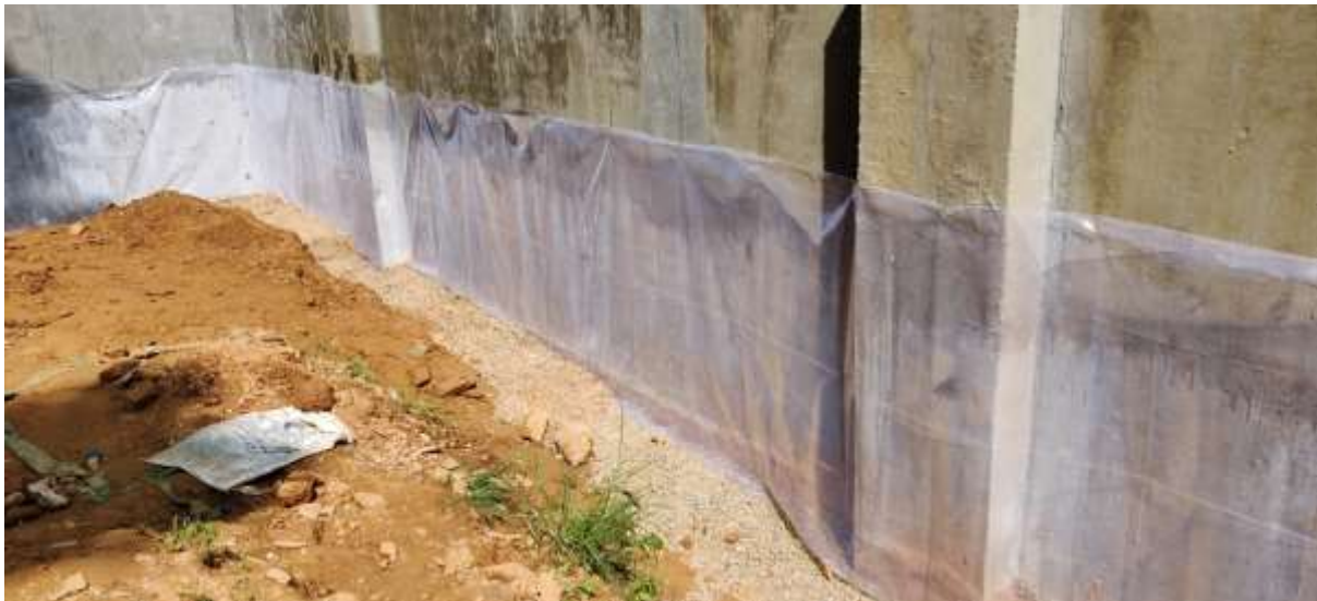
Picture 18: Laying of 500micron Plastic sheet over waterproofed RCC wall
