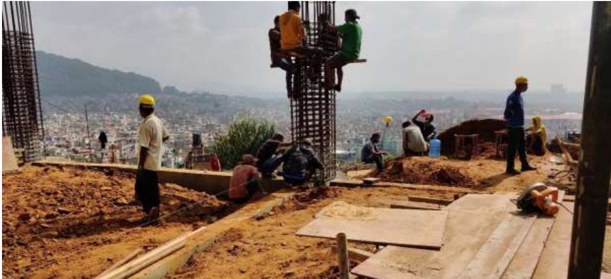
Picture 17: Rebar work for column at grid 5
