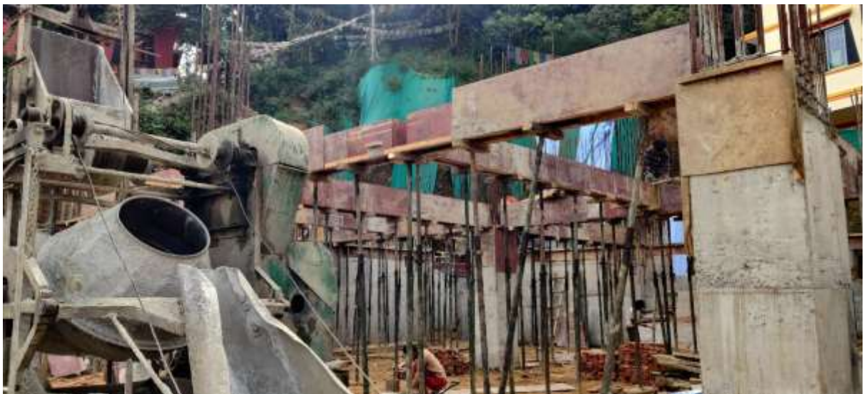
Picture 22: Formwork for upper ground floor level Beam
