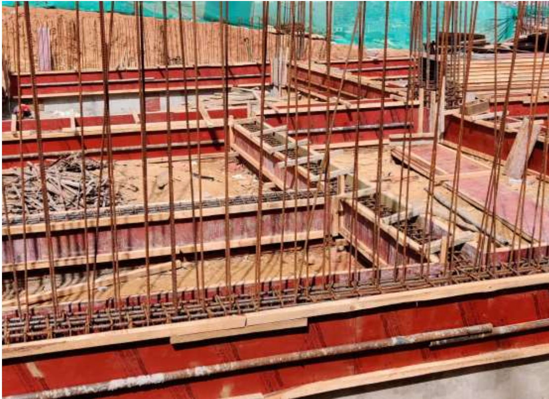
Picture 7: Formwork for Lower level Plinth Beam from Grid 1 to Grid 5
