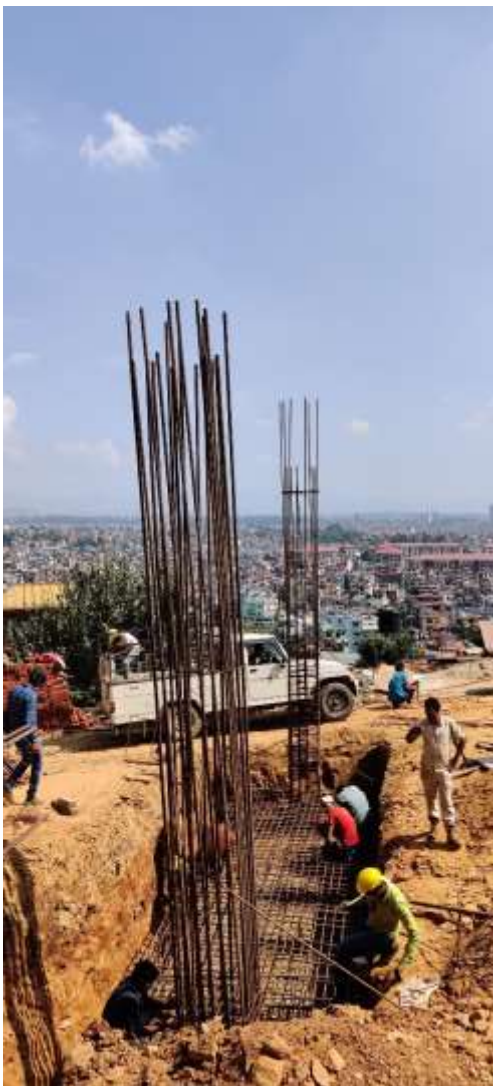
Picture 28: Rebar work for Foundation CF3
