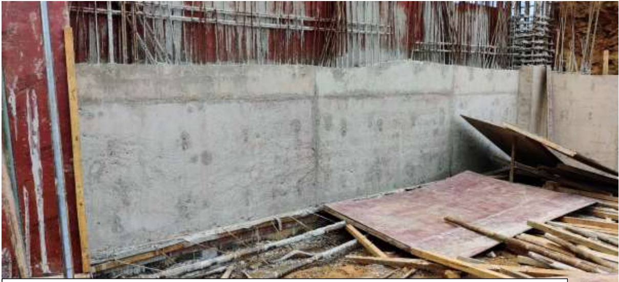
Picture 12: Shear wall after removal of formwork
