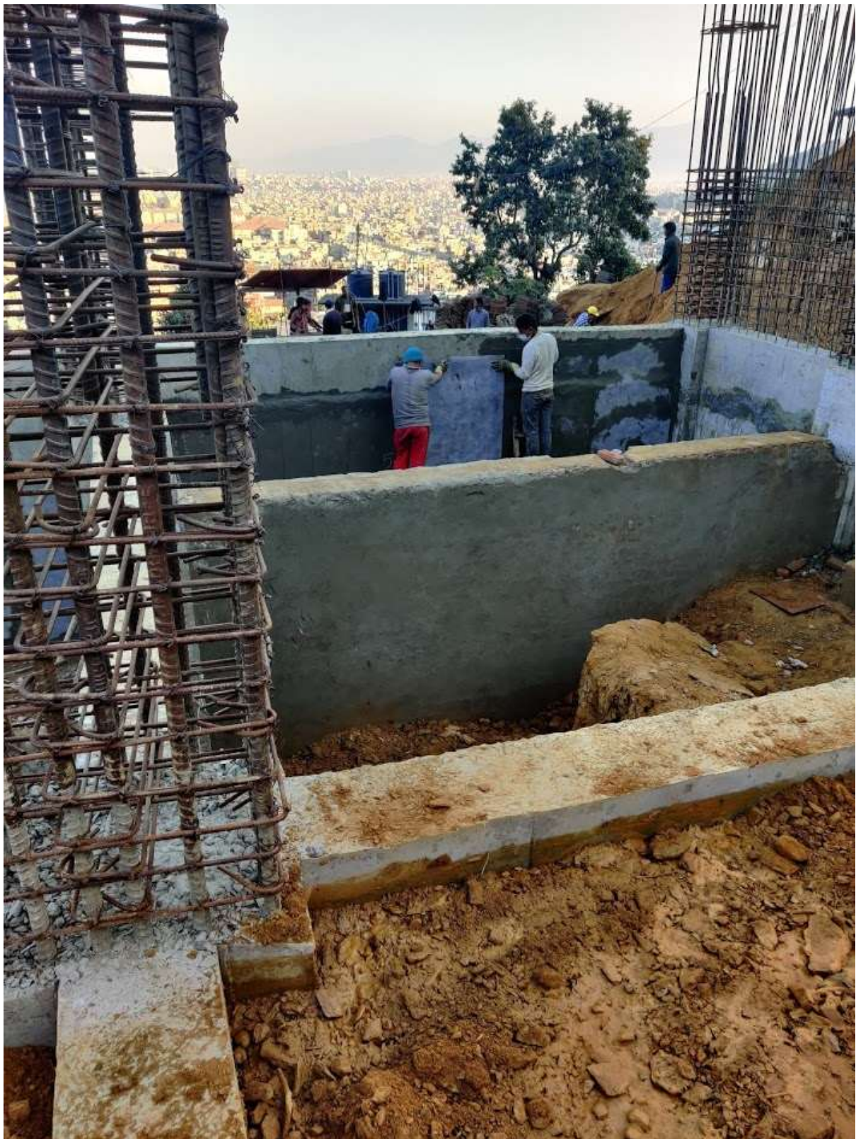
Picture 42: Laying of Membrane Sheet for water proofing
