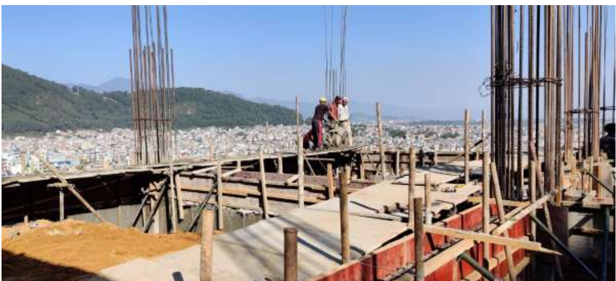
Picture 36: Concreting of lower ground Plinth Beam from grid 5 to Grid 8
