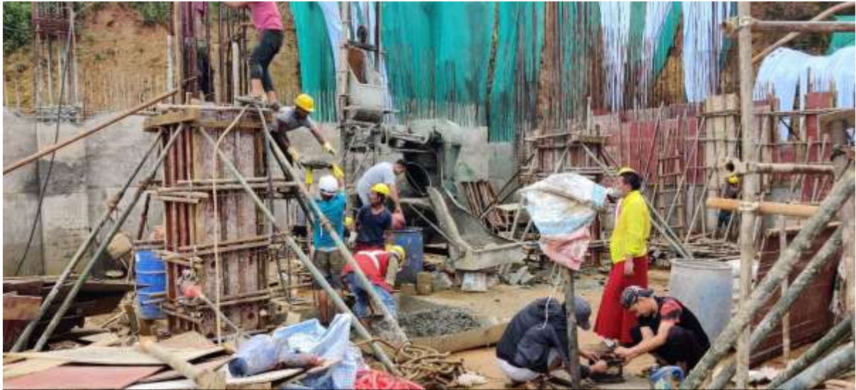
Picture 15: Concreting of Lower Ground floor Column
