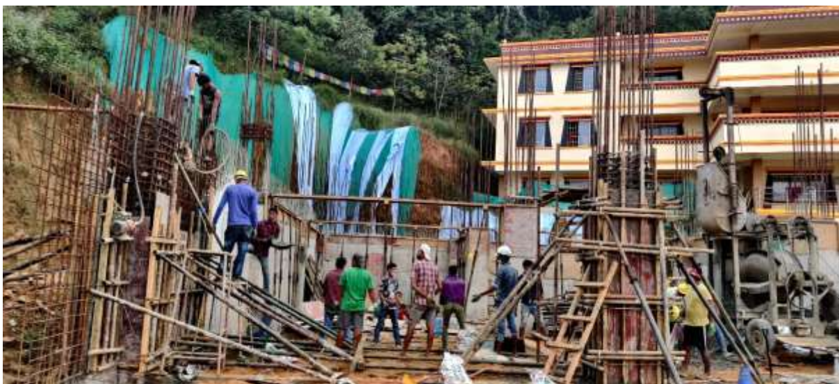
Picture 19: Concreting of Columns of Lower ground floor of Grid 5
