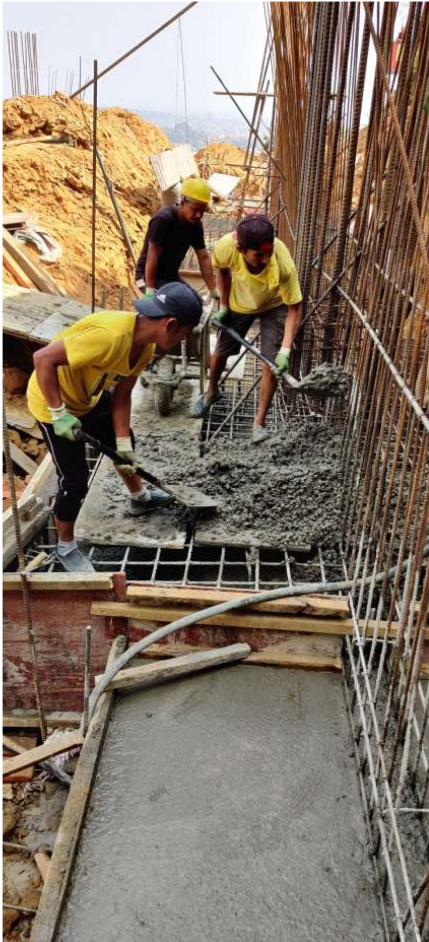
Picture 30: Concreting of Upper Ground level foundation
