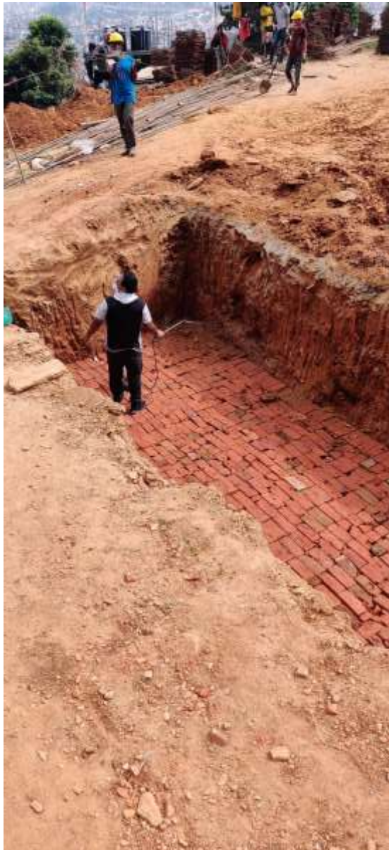
Picture 24: Spraying of Anti-termite at foundation CF3
