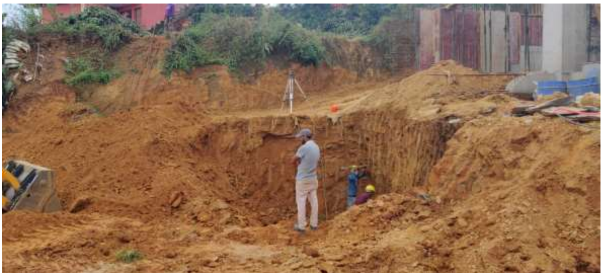
Picture 23: Excavation of foundation of lower ground floor level
