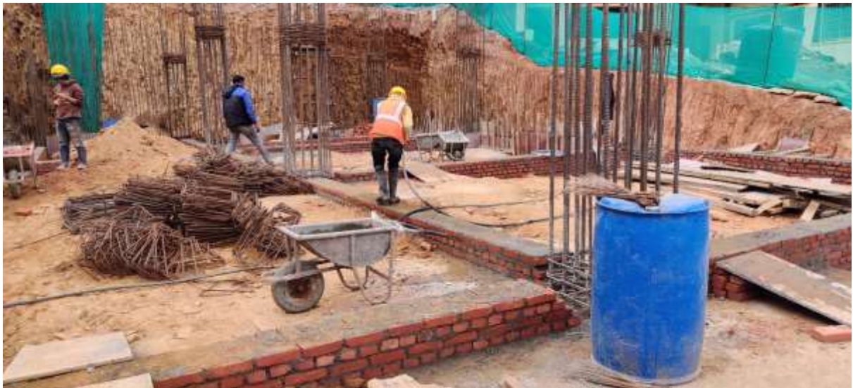
Picture 2: Brick Masonry work at Sub-structure of Grid 1 to Grid 5
