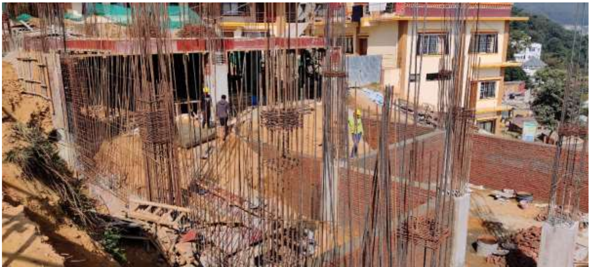
Picture 35: Brick Masonry work at lower ground level upto plinth level
