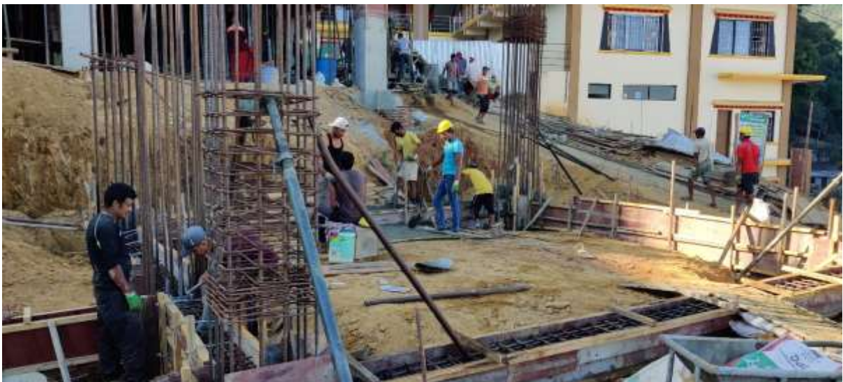
Picture 32: Formwork for lower level foundation beam
